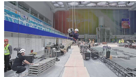
ロープが完全に張るまでゆっくり持ち上げること Lift slowly until the rope is fully straightened
